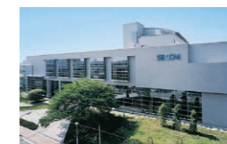
Mitaka Nisshin Building (former research laboratory)
