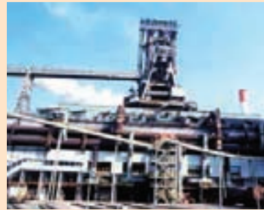
for steel & iron-making (Blast Furnace)
