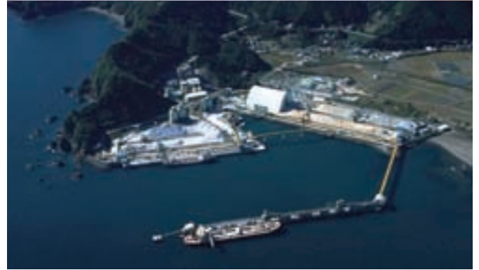
Torigatayama coastal facilities
