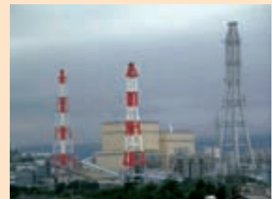
for flue gas desulfurization (thermal power station)
