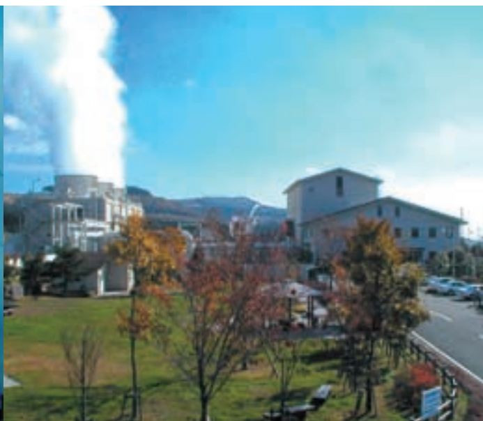
Ogiri Power Station
