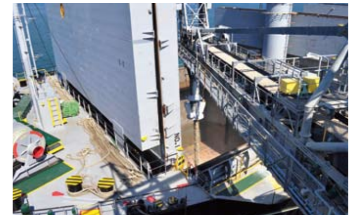
Loading limestone from the ship loader
